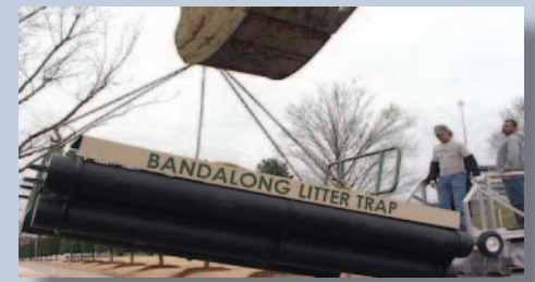
Employees installing Bandalong in Little Rock, AK in late February 2011
